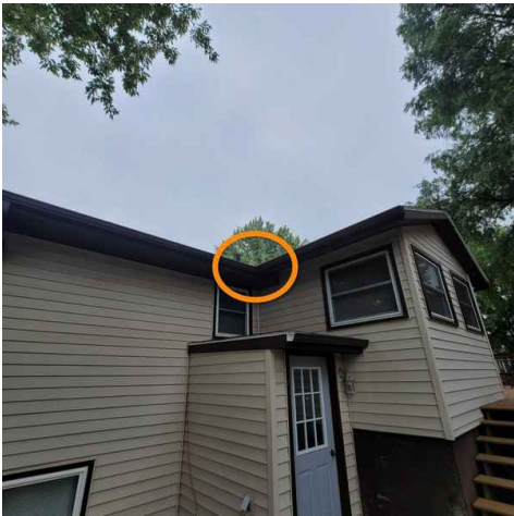
debris in gutters will prevent proper drainage
