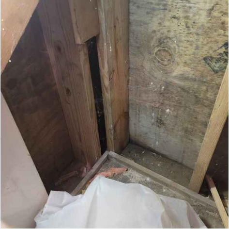
staining and signs of moisture witnessed
