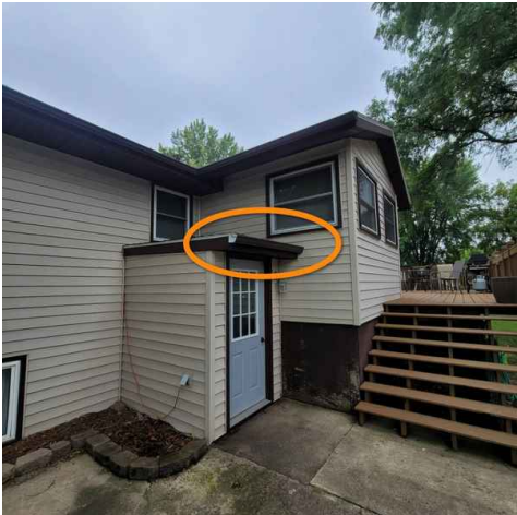
missing downspout allows water to spill next to the foundation - evidence of moisture at wood foundation noted at this area
