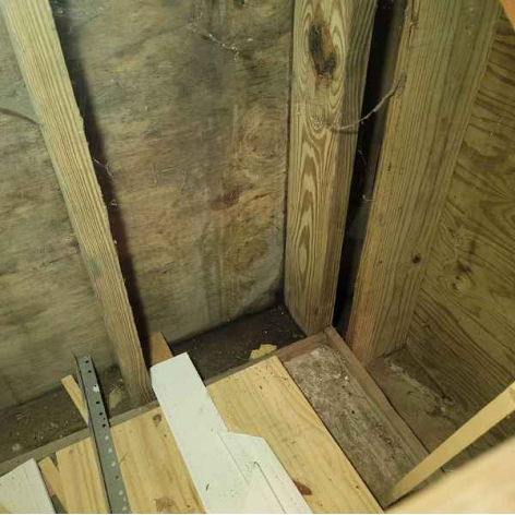
staining and signs of moisture witnessed
