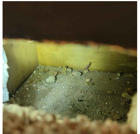
no staining/moisture witnessed at sill plate, base of stud, and treated plywood
