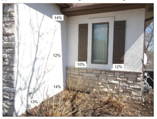
(2) The stucco is installed below grade or within six inches of grade. This can result in several problems including moisture wicking up from the soil, moisture entering the walls from above being unable to drain, and insects entering the wall from underground. Consider having the stucco trimmed to six or eight inches above grade and installing a weep screed for better drainage.
