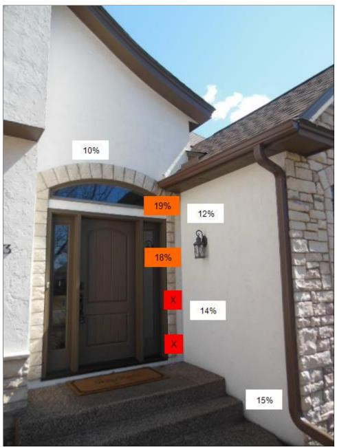
(2) Some kickout flashings were installed improperly and have the potential to allow for moisture intrusion. Have them properly re-installed.
