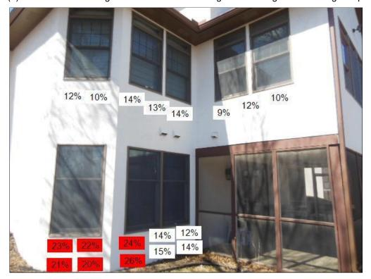
(2) Sprinklers to close to the stucco walls. Monitor or repair.
