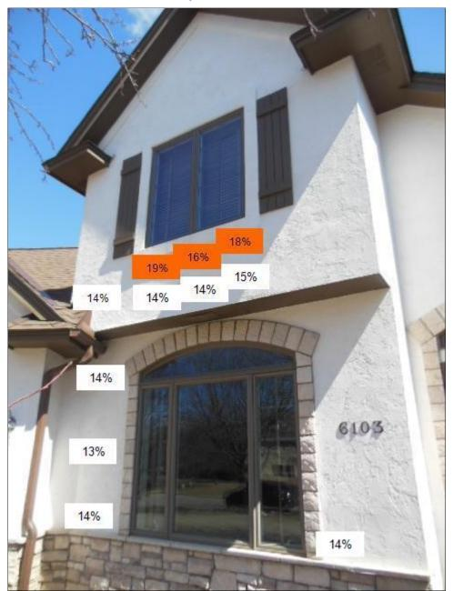
(2) The shutters are installed in an unsatisfactory manner by screwing through the shutters into the stucco. The installation of the shutters should be modified to provide better protection from possible moisture intrusion. Clip-on brackets are a better option; these brackets attach to the stucco cladding, are sealed, and then the shutter is snapped on.
