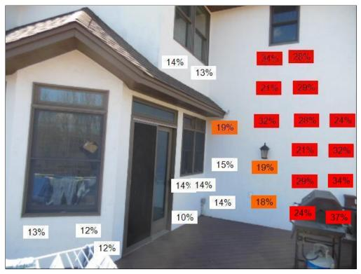
(2) Existing kickout flashings appear to be properly installed but are showing signs of high moisture intrusion. They may need to be re-installed, or if they were recently installed the affected areas may not have had adequate time to dry.
