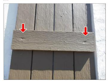
(3) The moisture readings in red were at 20% or higher indicating active leaking and possible structural damage.
